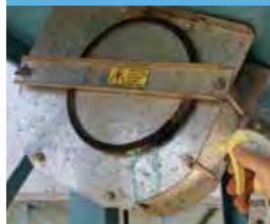
If the half-life pressure test is less than five minutes on a new silo, or three minutes on an old silo, there is a leak. To find leaks, pressurise the silo again and use soapy water in a spray bottle to check for air leaks around seals.
