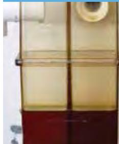
Oil relief valves are primarily fitted to protect the silo structure from damage due to air expansion and contraction when the silo is sealed during fumigation.
