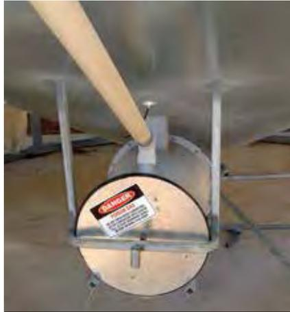
*Fumigation from below: Some silos are built with a chamber and passive (thermo-siphon) sealed recirculation system for applying phosphine from the bottom.*
